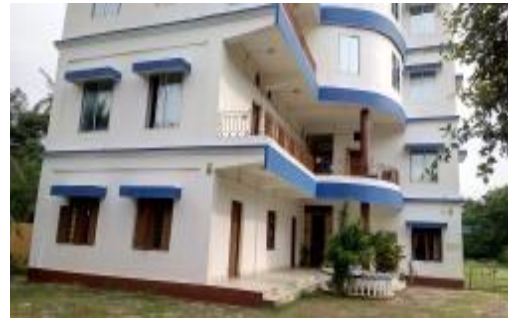
Balamuria Flood Shelter
