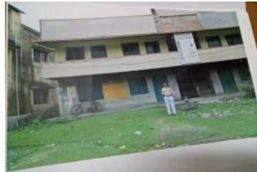
Kandapasara Flood Shelter
